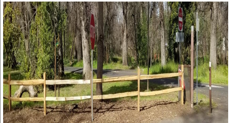
Figure 4: New split rail at Woodland Entrance
