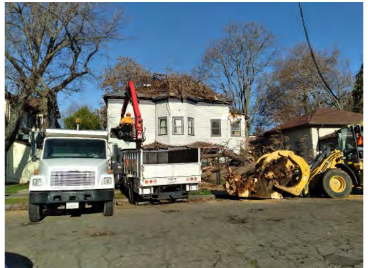
Figure 6: 4 th street cleanup operations.
