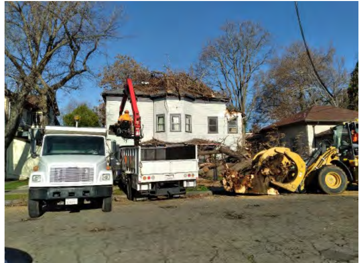
Figure 6: 4 th street cleanup operations.
