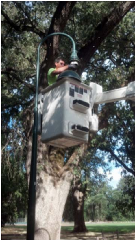
Ben Lepe of the City’s Public Works Department replaces old lights with LED’s that will reduce City maintenance and power costs and improve light quality and output.
