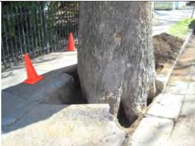
Before: Sycamore causing damage to sidewalk. Staff conducted a root collar investigation to check status of tree and health of root system.
