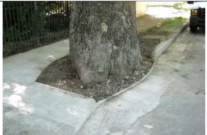
After: The tree was determined to have a healthy root deep roots, the sidewalk was repaired and widened to give a little more room for the tree.
