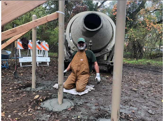
Figure 7 New Chin up Station install
