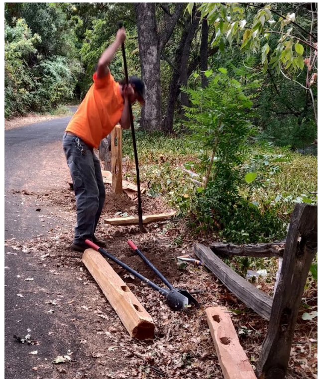
Figure 4 Split rail repair
