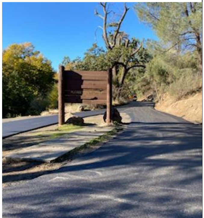
Figure 4-Upper Park Road Repaving
