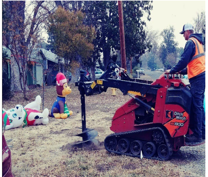
Figure 2 Contractor auguring planting spots in various locations around the city.
