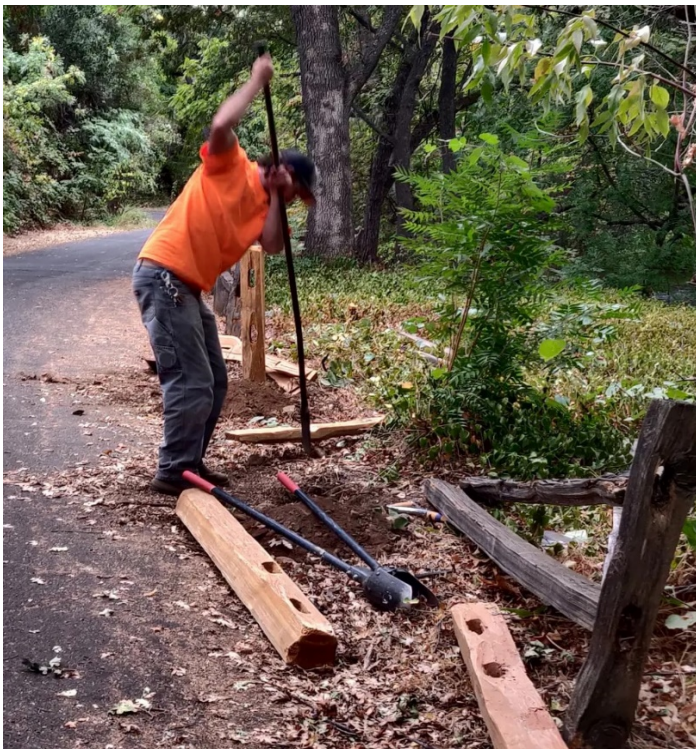
Figure 3 Split rail fence repair
