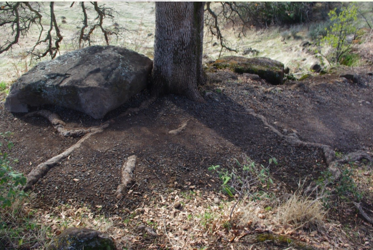
Once finished some trail work is subtle and many visitors are not aware that anything had been done. Soil and rock was brought in to protect the roots of this tree and minimize erosion
