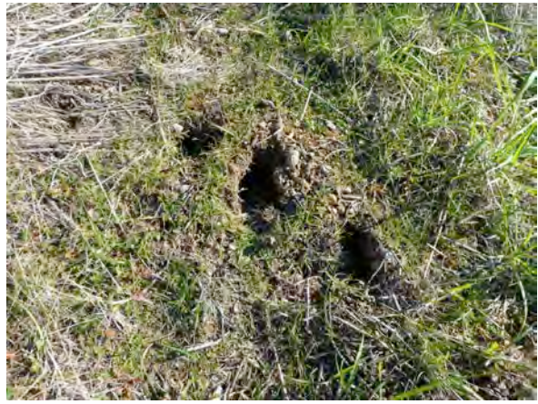
Photo 2: Rodent burrows and torn landscape fabric along western slope of landfill area.
