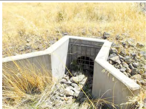
Photo 12: The catch basin outlet does not appear to be clogged.
