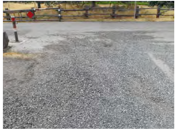
Photo 2: Gravel accumulating on Upper Park Road from the Horseshoe Lake parking lot.
