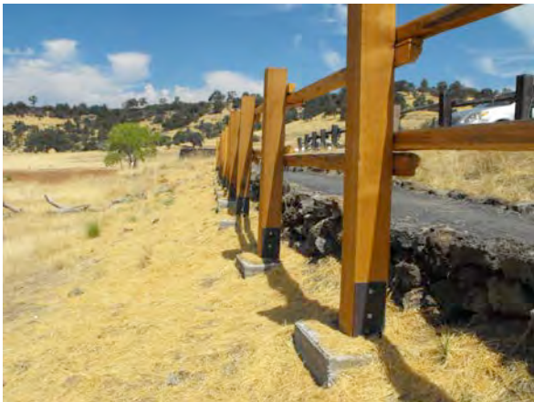
Photo 3: Newly installed fence along the west end of the containment cell.
