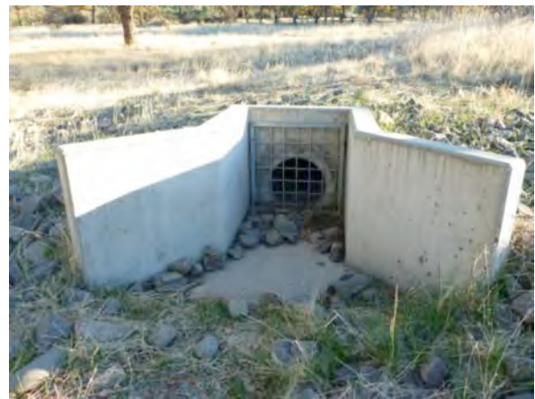
Photo 4: Pipe outlet looks clean and clear of debris.
