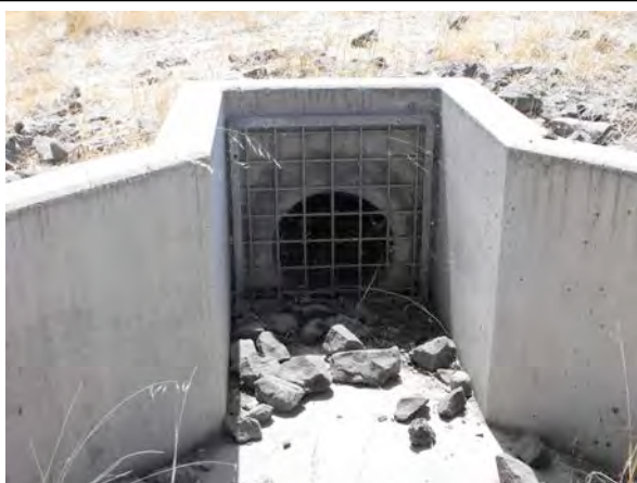
Photo 11: The catch basin inlet does not appear to be clogged.
