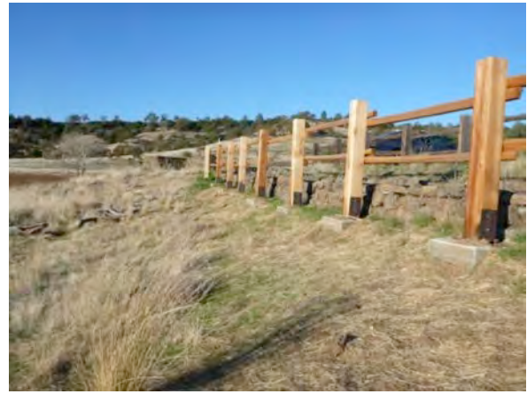
Photo 2: The new fence and trail have greatly reduced the use of pirate trails along the west slope of the containment cell.
