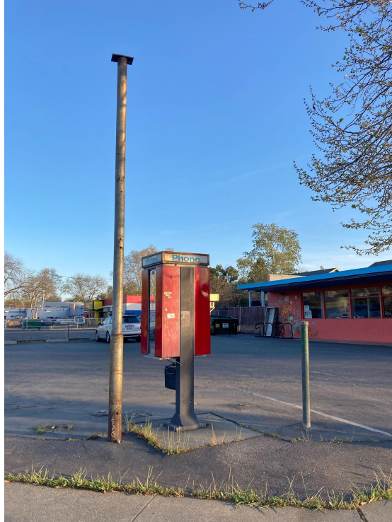
After removal of sign “can” and two bollards
