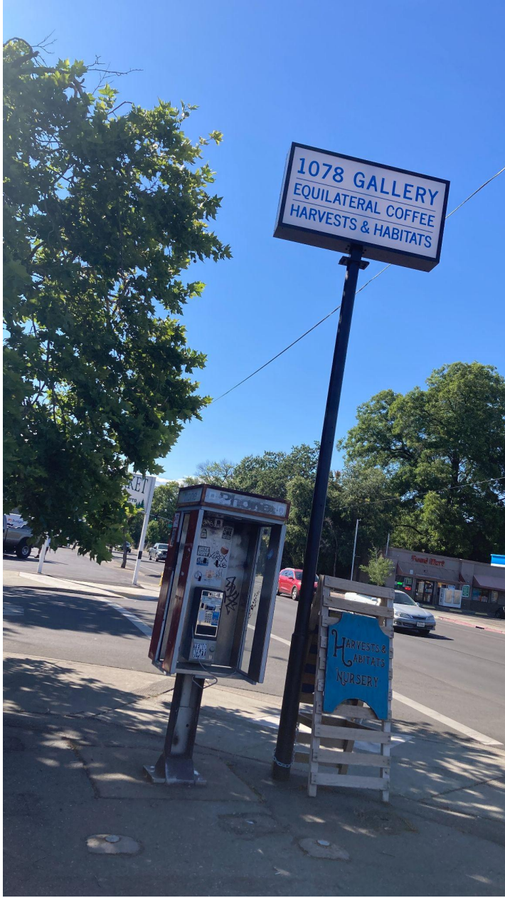
Completed sign installation
