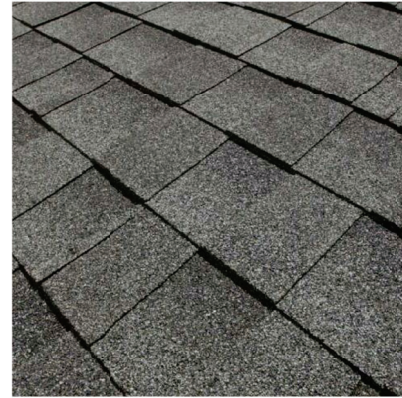
PAVILION ROOF ASPHALT SHINGLE ROOF
