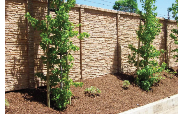
PROPERTY PERIMETER PRIVACY FENCE LAYERED STONE SOUNDWALL FENCE, 0% TRANSPARENCY 8' CONCRETE FENCE ALONG THE WESTERN PROPERTY LINE
