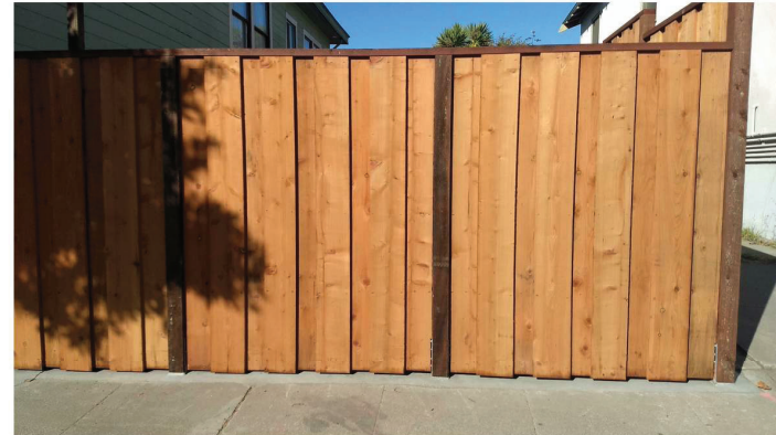
PROPERTY PERIMETER PRIVACY FENCE DECORATIVE WOOD, VERTICAL PATTERN, 0% TRANSPARENCY 6' WOOD FENCE ALONG THE SOUTHERN PROPERTY LINE
