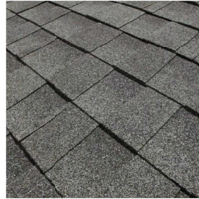
PAVILION ROOF ASPHALT SHINGLE ROOF
