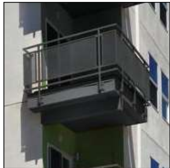
07 METAL BALCONY AND RAILING
