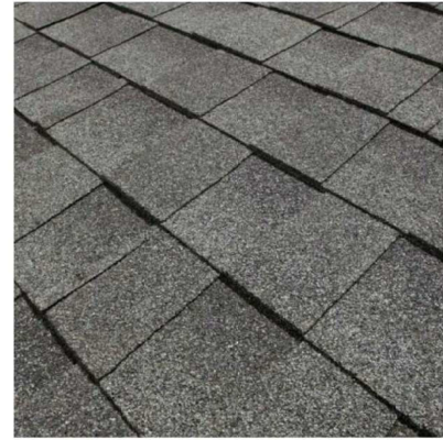
PAVILION ROOF ASPHALT SHINGLE ROOF
