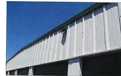
WALL MOUNTED STORAGE UNIT LIGHTING
