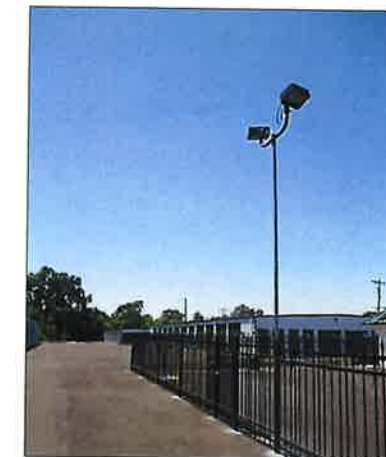
FREE STANDING SECURITY LIGHTING
