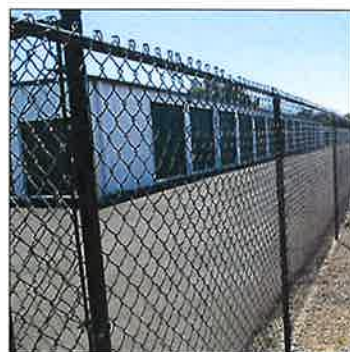
TYPICAL STORAGE UNIT SECURITY FENCING
