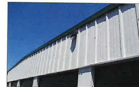
WALL MOUNTED STORAGE UNIT LIGHTING
