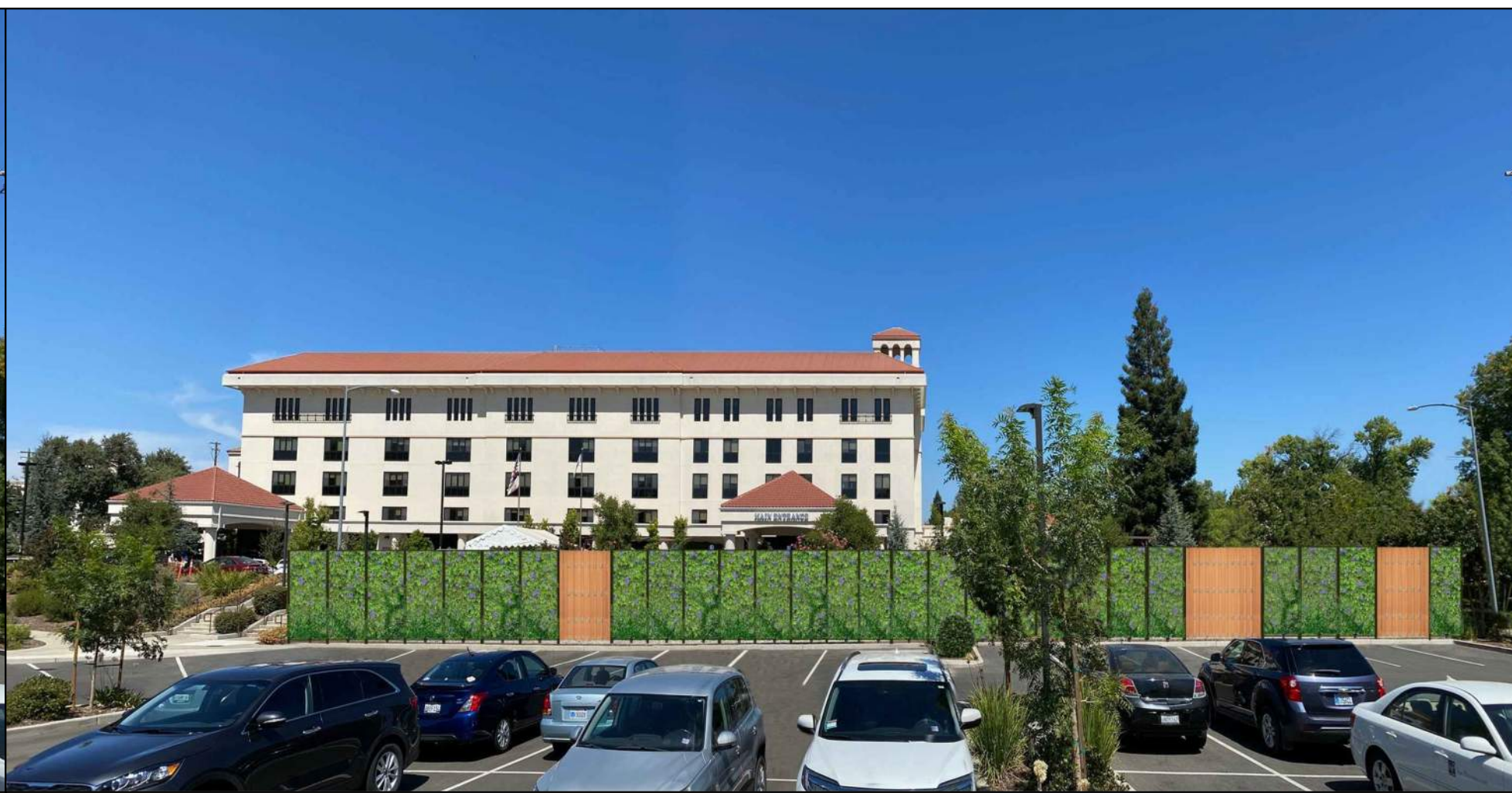
WOODEN GATES AND VINES AT INITIAL INSTALL WITH MESH MATERIAL ON INSIDE OF FENCE
