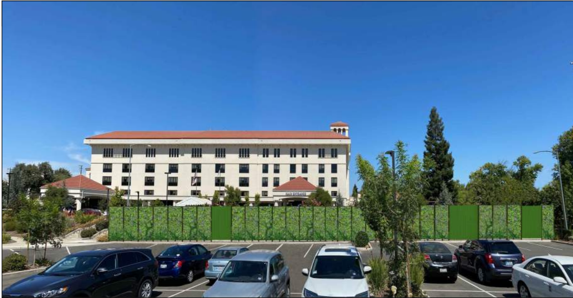
METAL PANEL GATES AND VINES AT INITIAL INSTALL WITH MESH MATERIAL ON INSIDE OF FENCE
