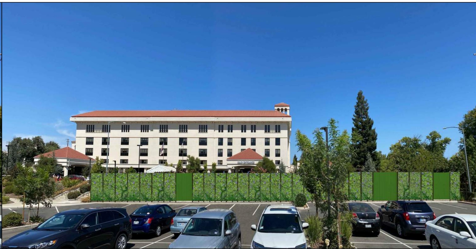
METAL PANEL GATES AND VINES AT INITIAL INSTALL WITH MESH MATERIAL ON INSIDE OF FENCE
