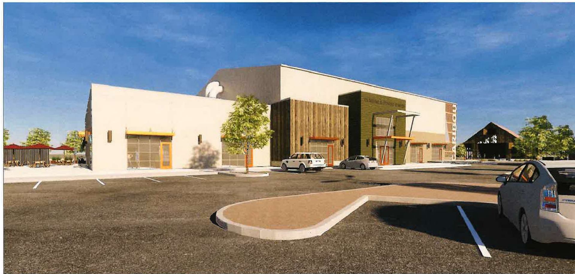
Facing Southeast View ( From Parking Lot )
