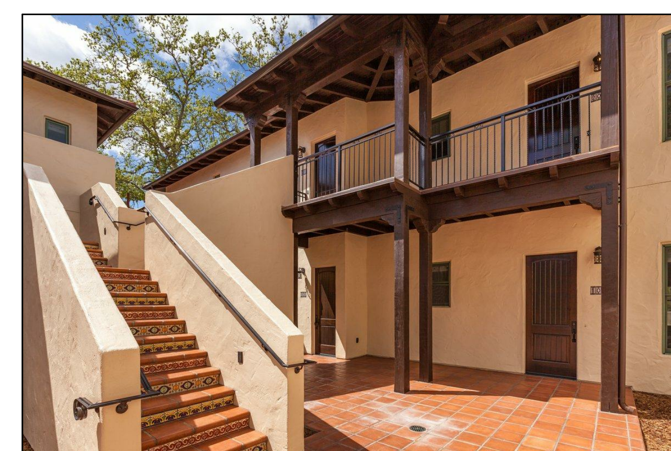
THE ARCADIAN - INTERNAL COURTYARD STAIR & WALKWAY
