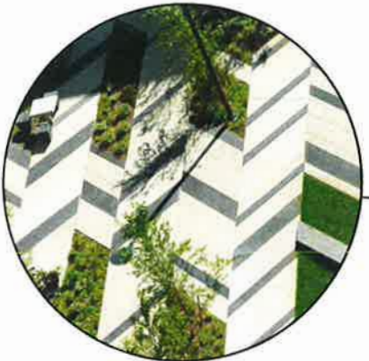
Plaza Paving Two toned shot blasted concrete
