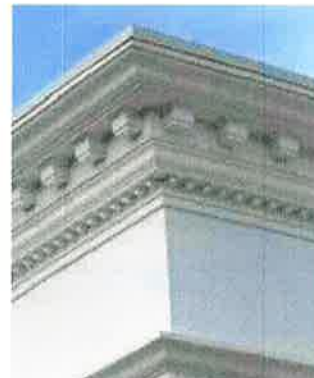
PRECAST LIMESTONE/GFRC CORNICE (PROFILE SIMILAR) HONED FINISH REFER TO ELEVATION FOR PROPOSED COLOR
