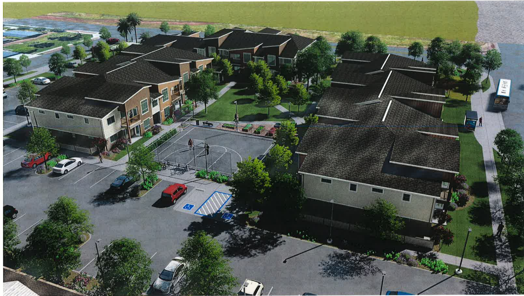
1 OVERHEAD VIEW OF COURTYARD LOOKING SOUTH
