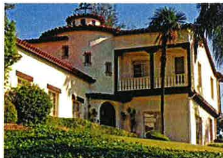
Bridgford House (1927) 401 Cannon Lane
