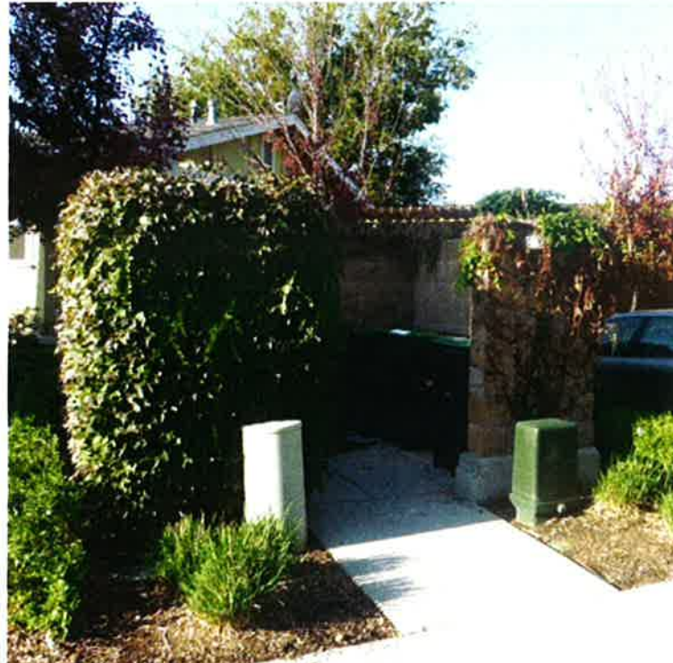
TRASH ENCLOSURE 6' tall concrete block wall trash enclosure landscaped with lilac vine.
