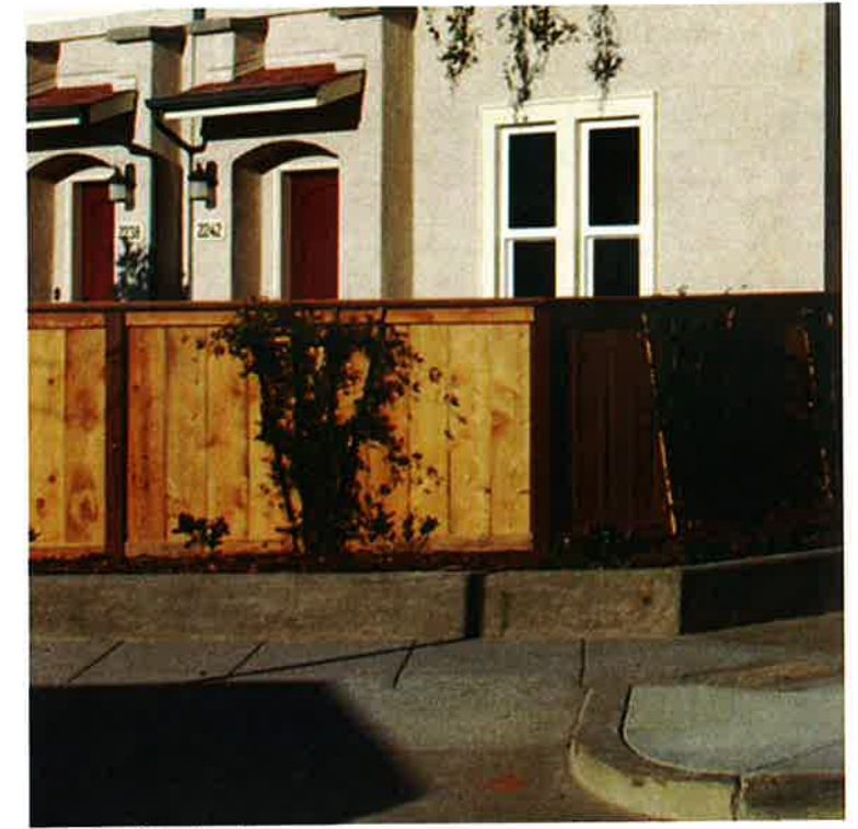
FENCE (Typical) 4' & 6' tall wooden fence with beveled cap and trim boards at top and bottom.
