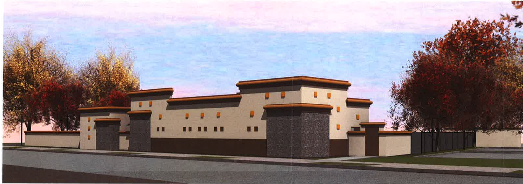
ALCOTT AVENUE SUPPORT BUILDING NORTH VIEW
