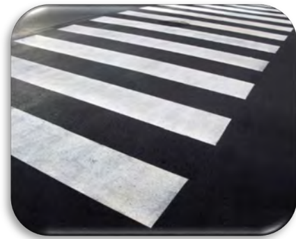
Exhibit 7. High-visibility or “Continental” Crosswalk markings improve pedestrian crossing visibility
