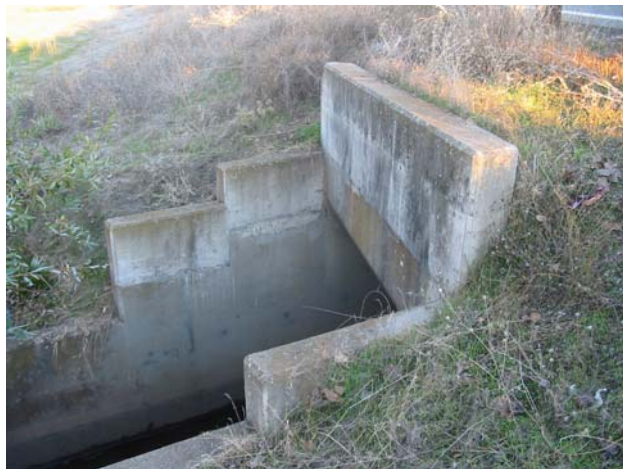
Photo 7. Downstream Headwall of South Fork RCB
