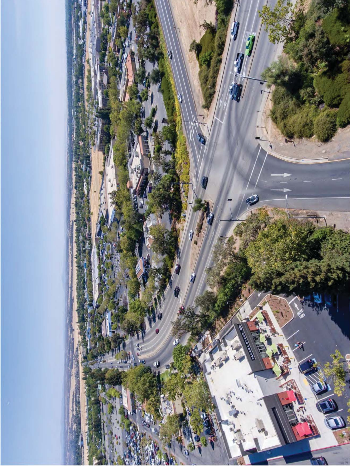
NB On-Ramp – Photo 3
