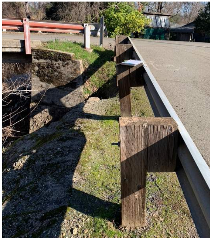
Photo 2. Treated wood posts at southeast corner of the bridge. 2/6/2020.
