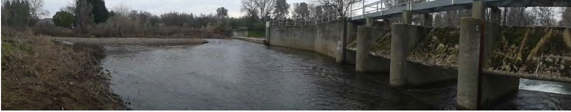
Figure 3: Little Chico Creek diversion structure; sluice gates (near) and Little Chico Creek Diversion Channel diversion weir (distance).
