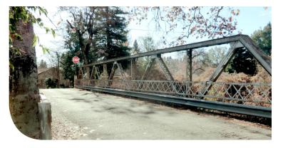
The existing bridge is an 86-foot long, single-span, steel Warren pony truss bridge. The bridge is structurally deficient and functionally obsolete for the following reasons:
