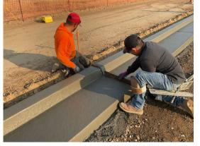
On Bruce Road between Skyway and E. 20th Street, the road is beginning to take shape with the installation of concrete curbs and gutter. The underground utilities have been substantially completed, making way for final paving to commence later this month.
