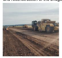
involved the removal of asphalt and excavation of the roadway between Skyway and E 20th Street in preparation for the new Roller Compacted Concrete (RCC) roadway. A new storm drain trunkline was installed from Fremont Street to Bruce Road along what will be the future "Webster Road", as well as completion of a new storm drain installed along Bruce Road between Skyway and E 20th Street. At the new bridge location between Concord Ave and Banner Peak,
