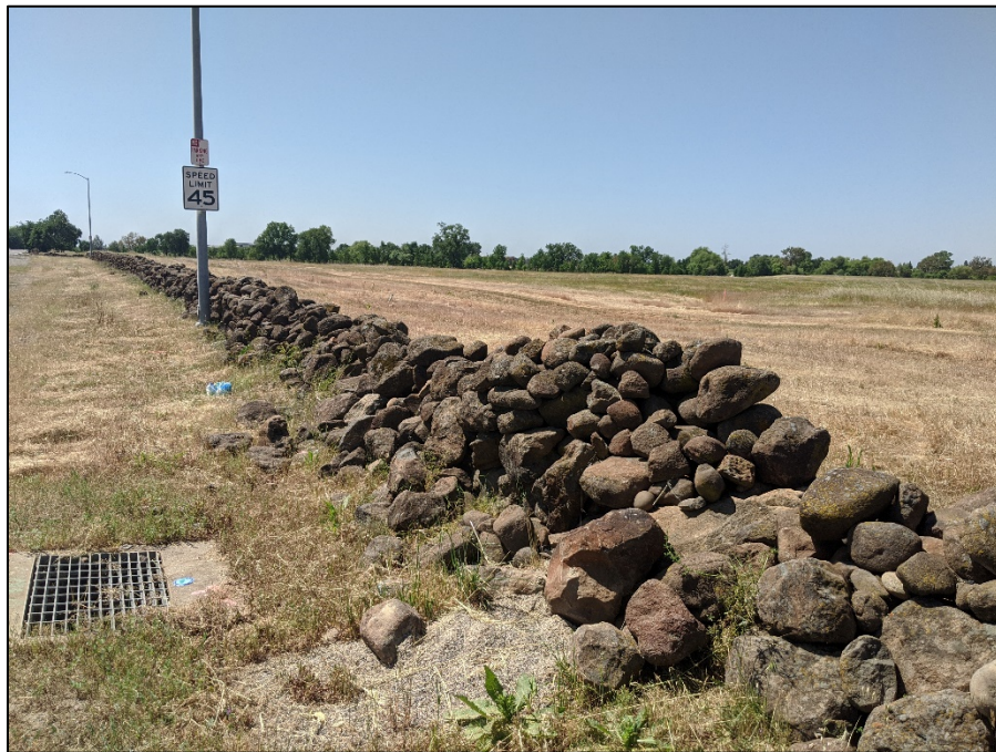
Photo 2. Overview of CA-BUT-1071H (Bruce Ranch Stone Fence) and Bruce Road ROW, view south, photo taken November 4, 2019.
