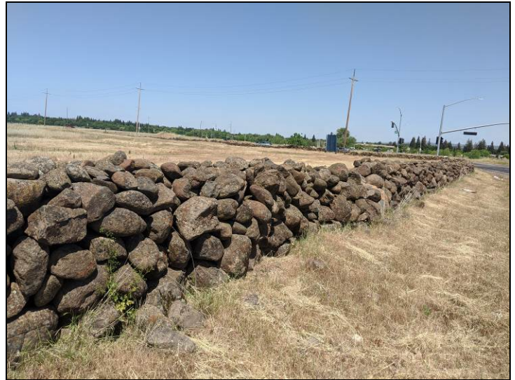
Rock wall, view NW towards Humboldt Road, 5/1/2020, Photo_002
