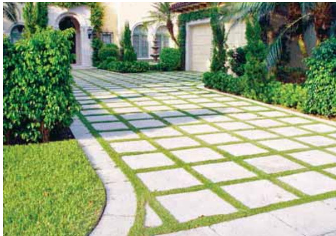
Residential pervious paving.
