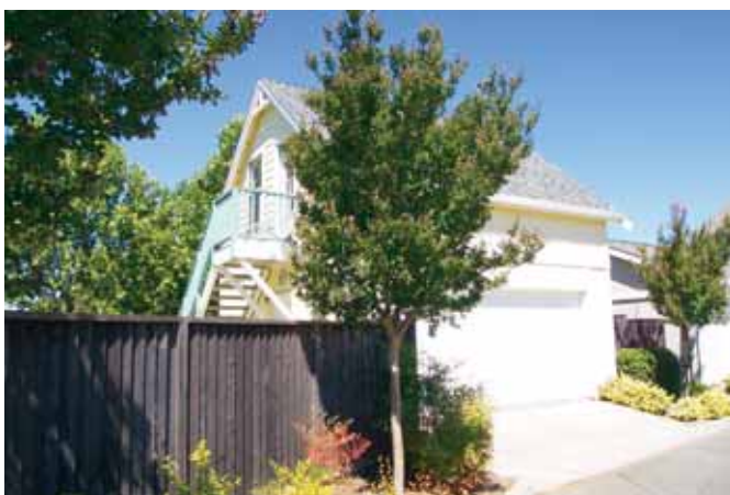
Second dwelling unit to the rear of the primary dwelling.
