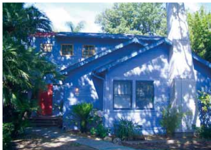
New construction respecting the original dwelling.
