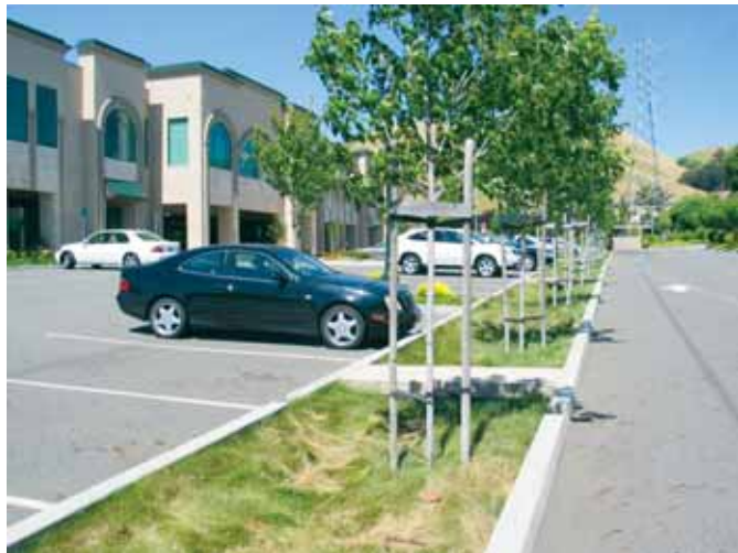
Grassy bio-swale to increase stormwater retention.
