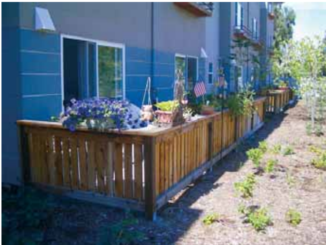
Low residential fencing providing privacy and visibility.
