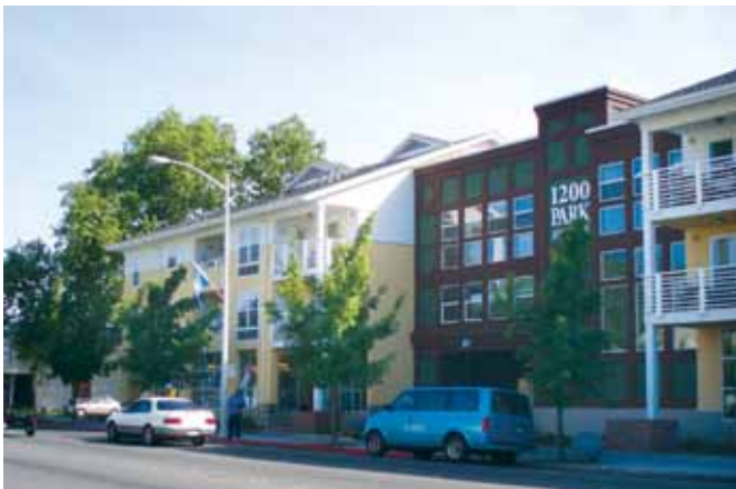
Existing 3-story senior housing in SW Chico, CA.
