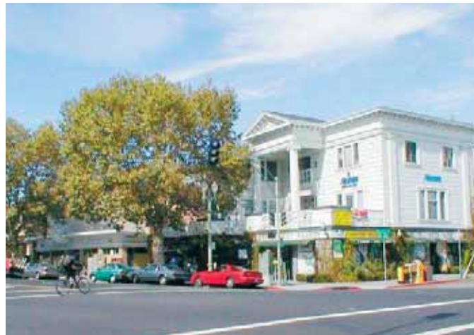
Mixed-use building helping to define the street as a public space, Adams Point, Oakland, CA.
