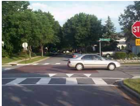
Figure 5-10-J. Speed Platform (Raised Intersection).
