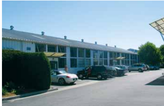
Live/Work housing in Santa Cruz, California.
