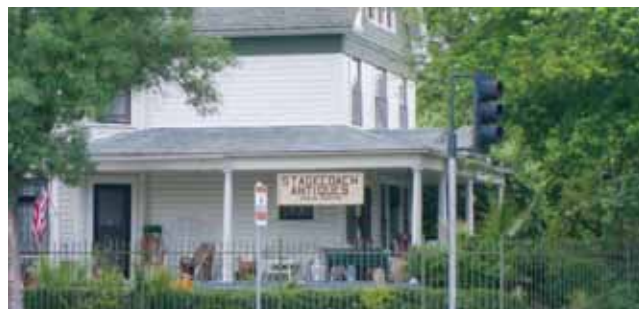
Commercial use in historical building on Park Avenue.
