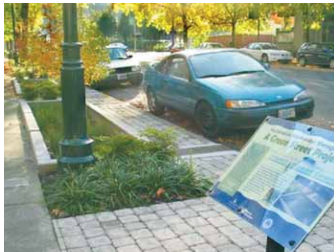
Green Street project in Portland, OR designed to capture street runoff.
