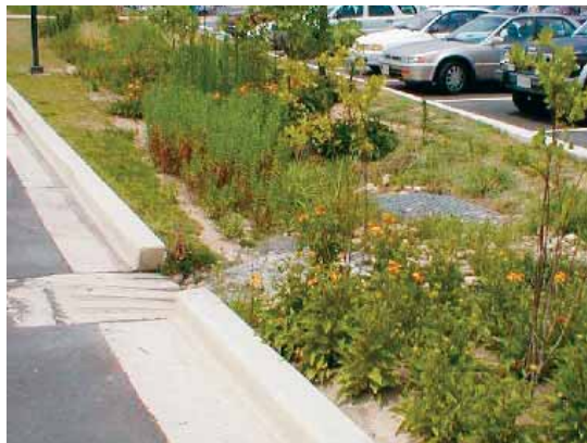
Grassy bio-swale with perforated curb.
