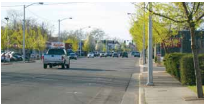
Streetscape improvements on Park Avenue north of 20 th Street.
