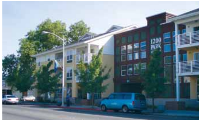
The 1200 Park Avenue Senior Apartments and the street improvements around it were built following the Vision Study's design guidelines.
