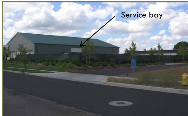
DG 6.1.22- Service bay located at the rear of building and accessed from rear driveway
