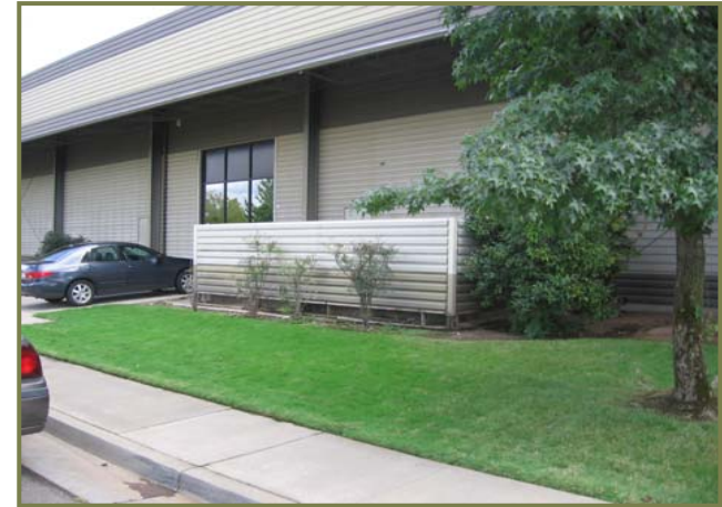
DG 6.1.49- Architectural screen compliments building
