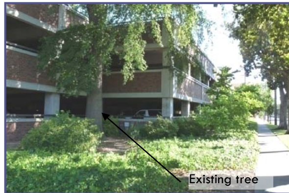
DG 5.1.41- Priority was given to the existing tree during the design phase
