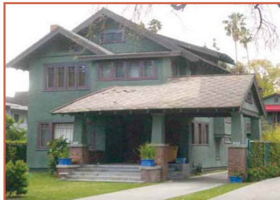
DG 4.1.61- Carport is designed with respect to the character of the house
