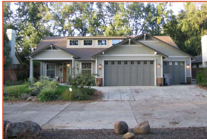
DG 4.1.11 & 4.1.12 - Large front porch is not dominated by attractive style and color of garage doors - Recommended
