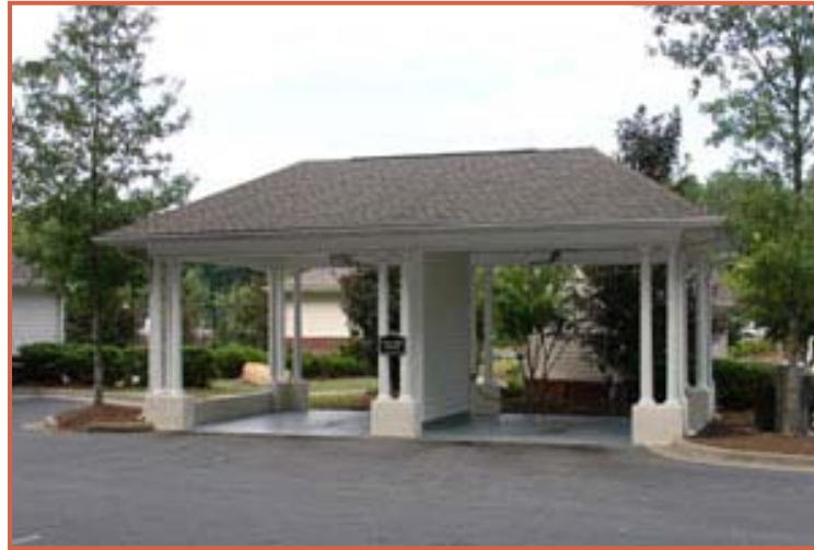
DG 4.1.54- Common vehicle wash area
