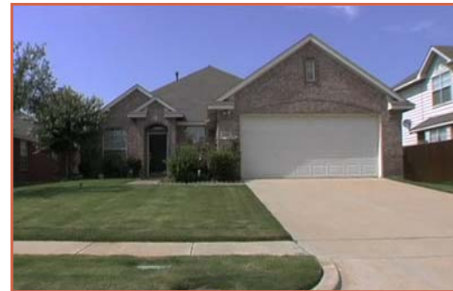
DG 4.1.61- Not Recommended - Garage is set in front of house and dominates the front façade
