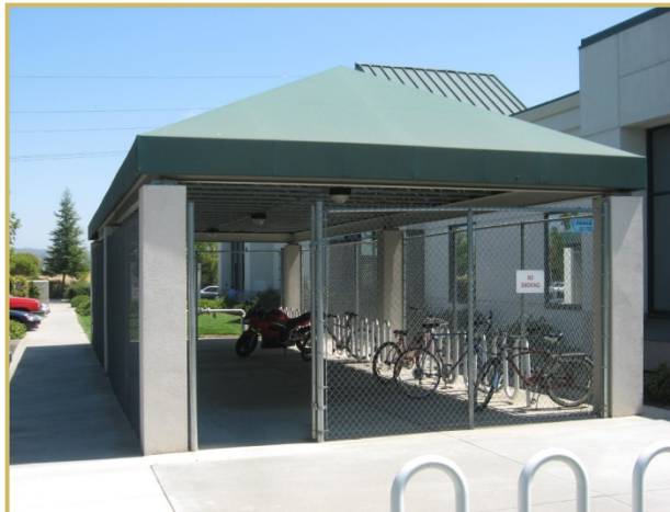
DG 2.1.31 and 2.1.32 - Covered and secured bike parking
