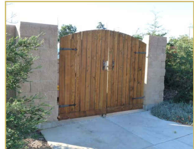
DG 2.1.37- Trash containers are concealed behind a well designed trash enclosure and landscape
