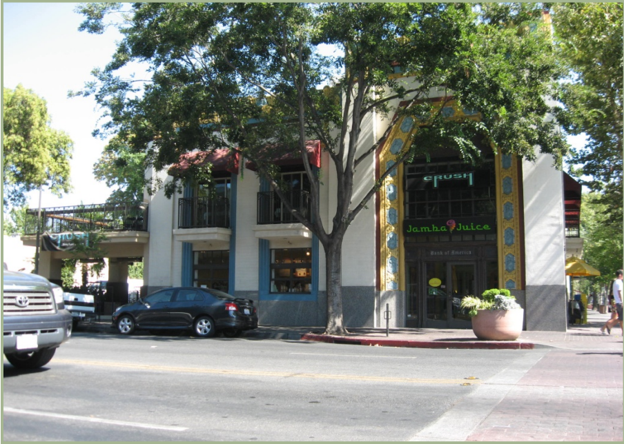
DG 1.3.69 & 1.3.73- Store front remodeled to reflect character of the past
