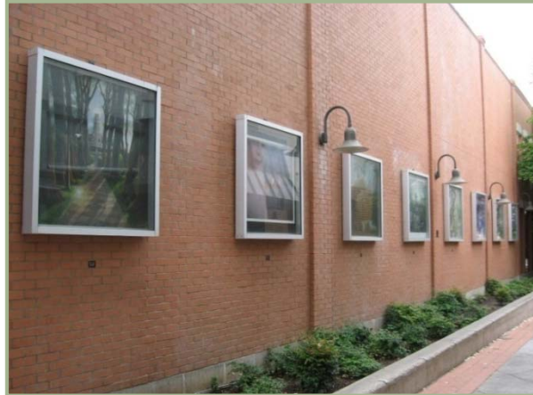
DG 1.3.31- Paintings enrich a public alley and add interest to a monotonous brick wall
