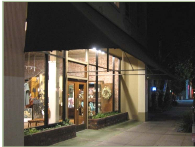
DG 1.3.56- Lighting provides security after hours
