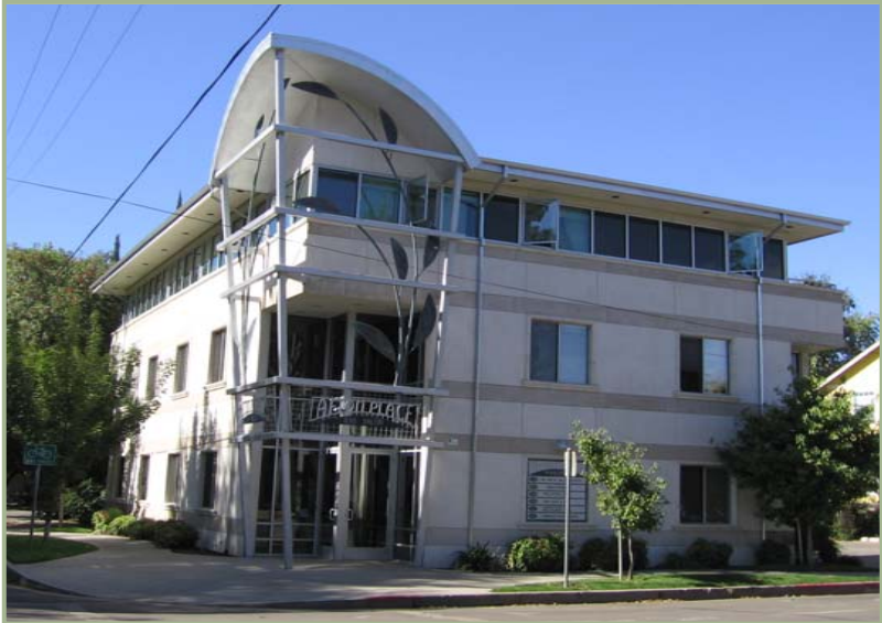
DG 1.4.11- Art and architecture blend for function and aesthetics, and to reinforce a sense of place
