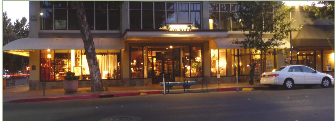
DG 1.3.56- Effective lighting creates a lively store front
