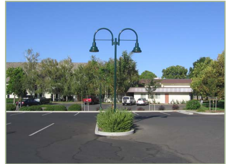
DG 1.5.15 – Architecturally styled with full cutoff fixtures
