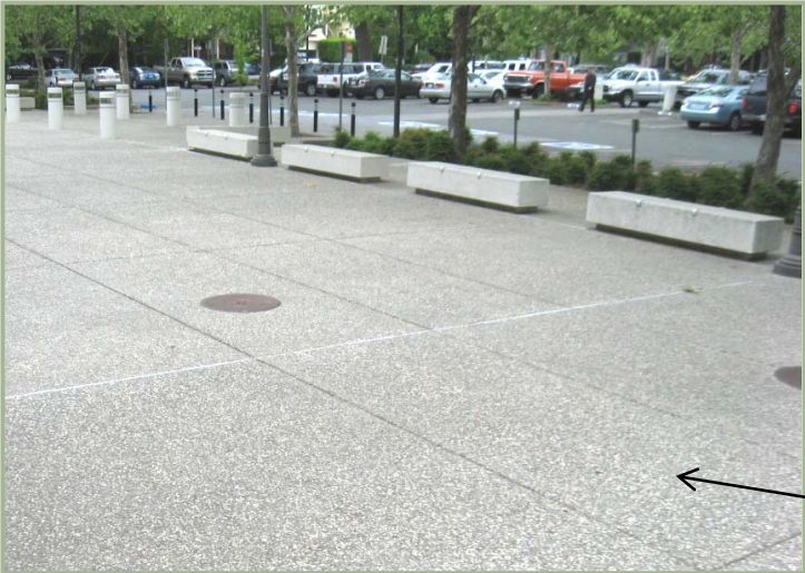
DG 1.3.43- Paving pattern at Chico Municipal Center
