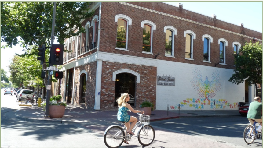
DG 1.3.98 Storefront consistent with adjacent historical character
