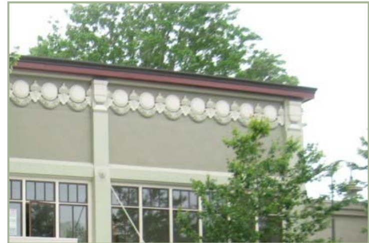
DG 1.3.76- Cornice detail
