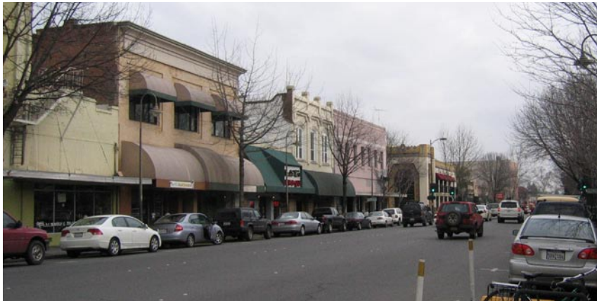
Existing 3-lane, one-way circulation on Broadway could be reconfigured to allow two-way circulation.
