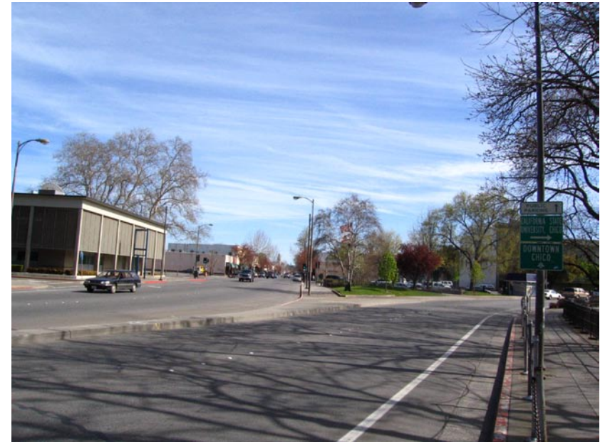
Current configuration at northern entrance to downtown
