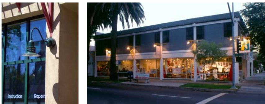
Figure D-13. Outdoor Lighting Mounted on Buildings.
