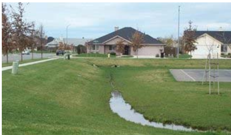
As shown above, Nob Hill Park will be a model for a new park and drainage facility in the western portion of the Plan Area
