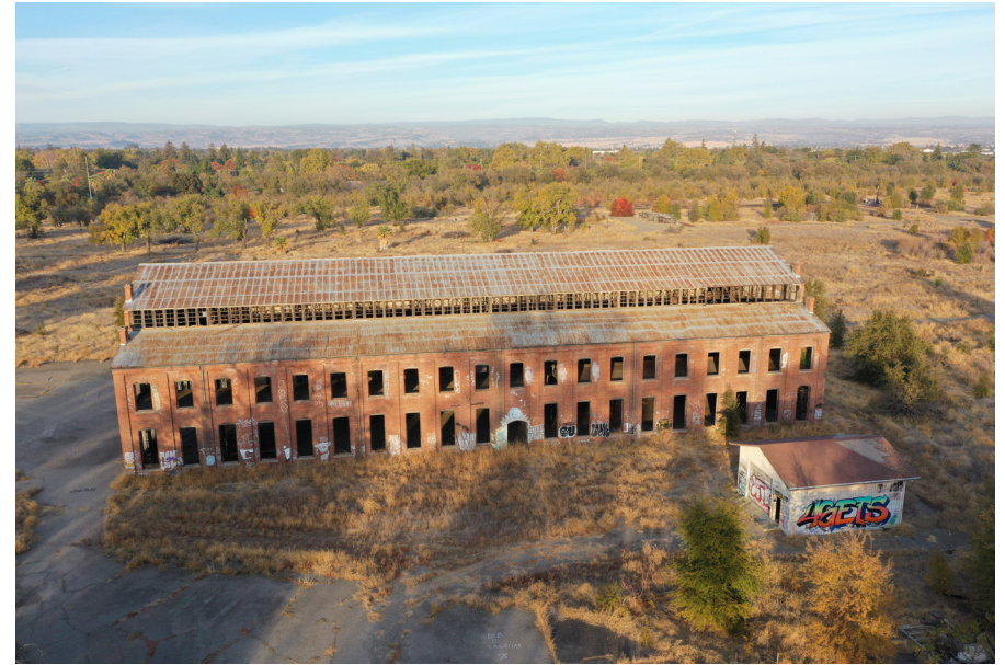
Figure 6.2 Existing site aerial
