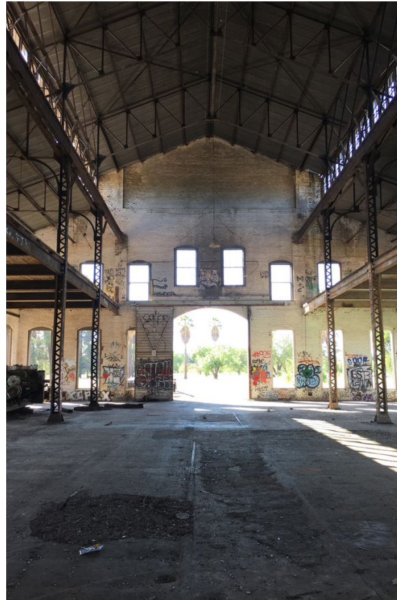
Figure 4.18 Interior view of the existing Engineering Building
