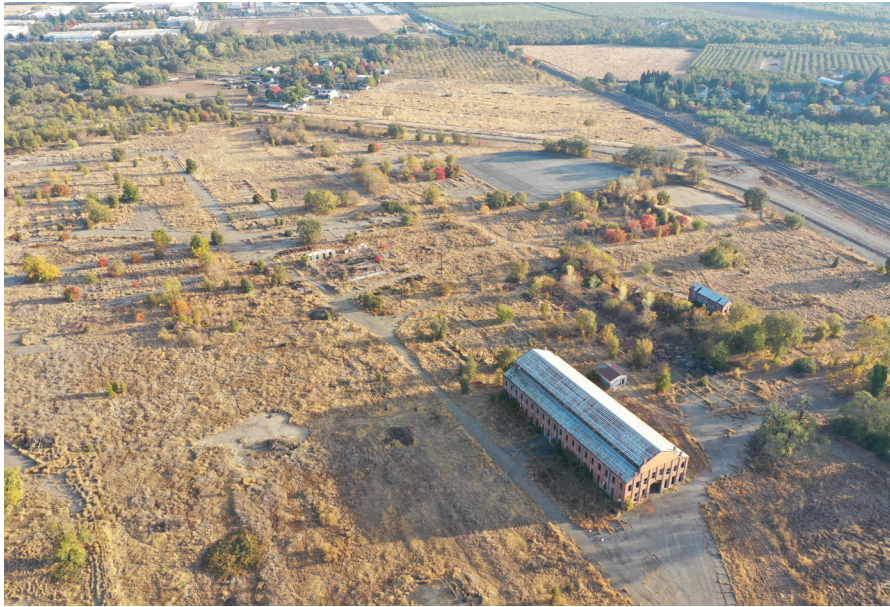
Figure 6.1 Existing site aerial
