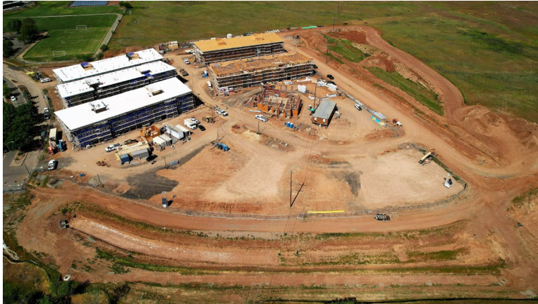
Photo courtesy of Sunseri Construction
