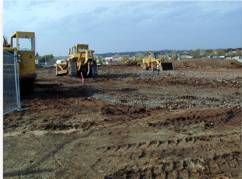
Subdivision grading in process
