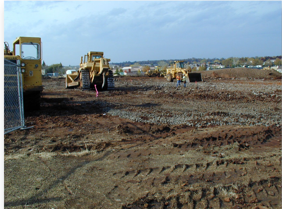
Subdivision grading in process
