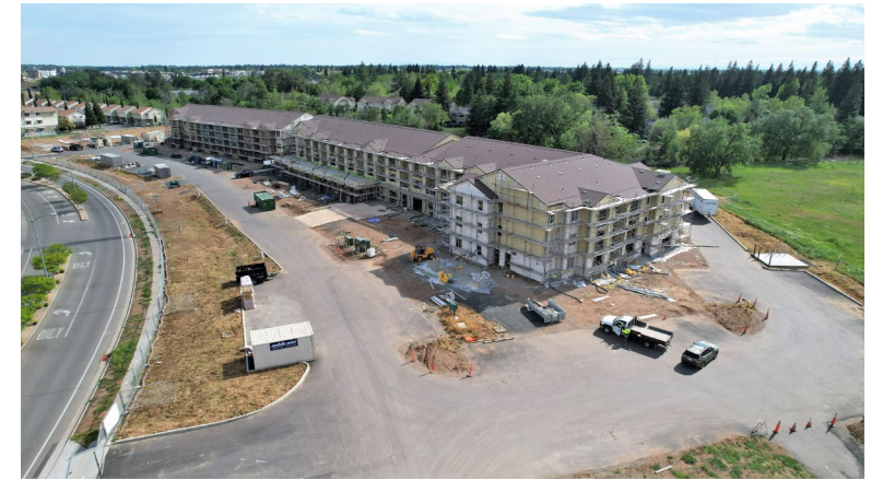
Photo courtesy of Sunseri Construction
