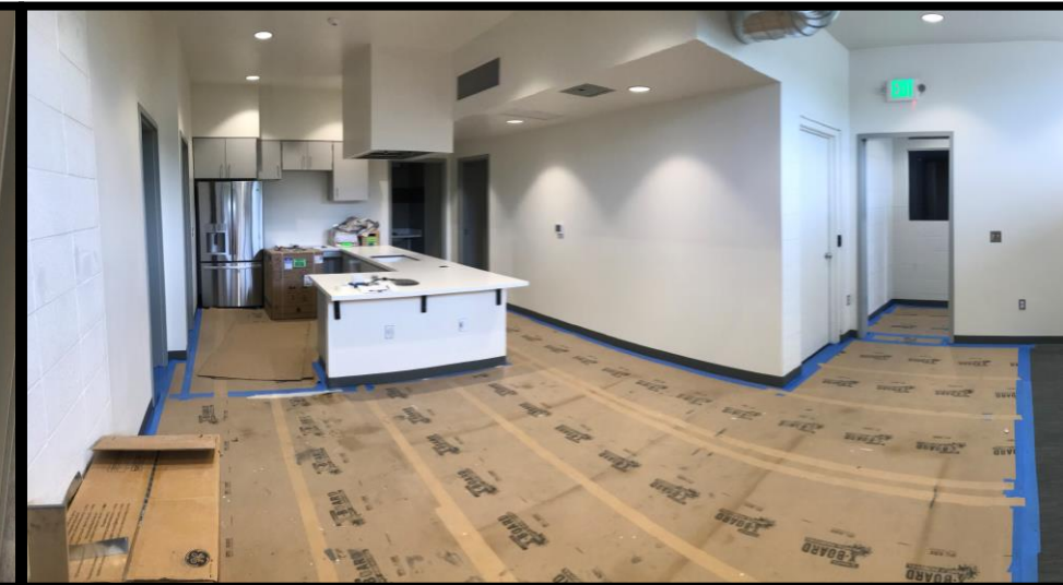
FS #1 Remodel – Phase 3
