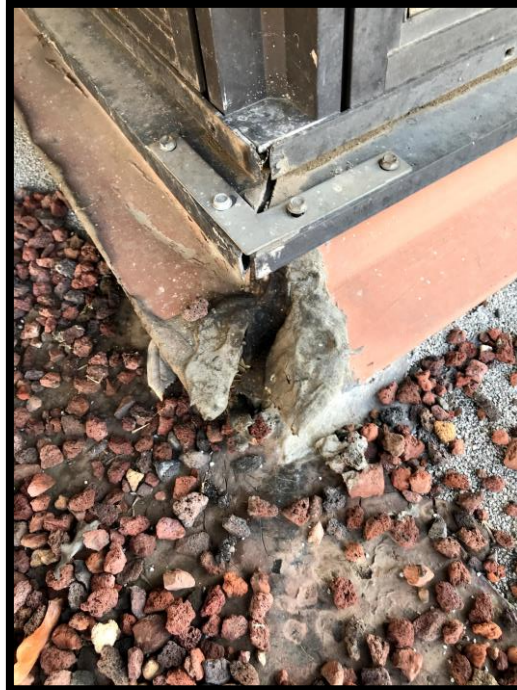
Council Chambers Window Frame
