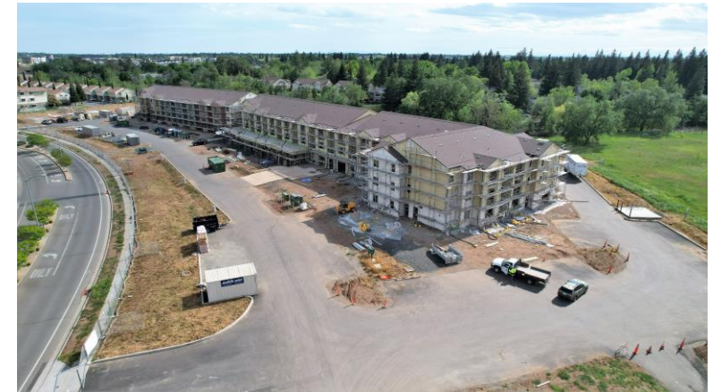
Photo courtesy of Sunseri Construction
