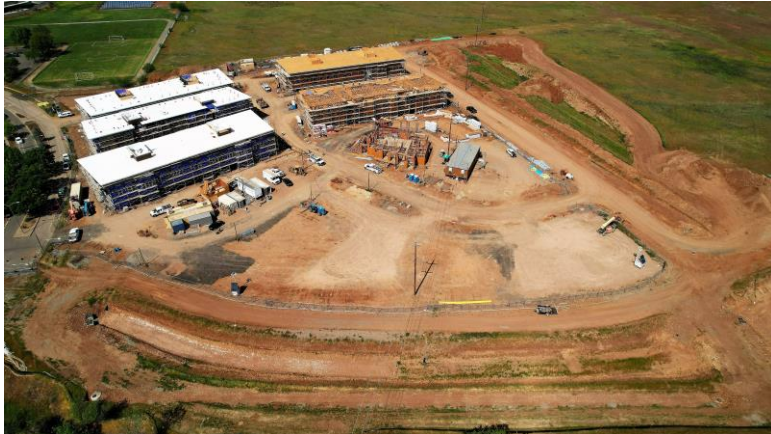
Photo courtesy of Sunseri Construction
