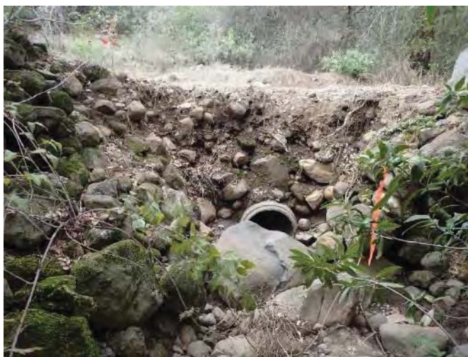
Figure 1. This stream crossing site is plugged by a boulder that dwarfs the concrete culvert inlet. The culvert is undersized for the upslope drainage area and was assigned a high priority for treatment.
