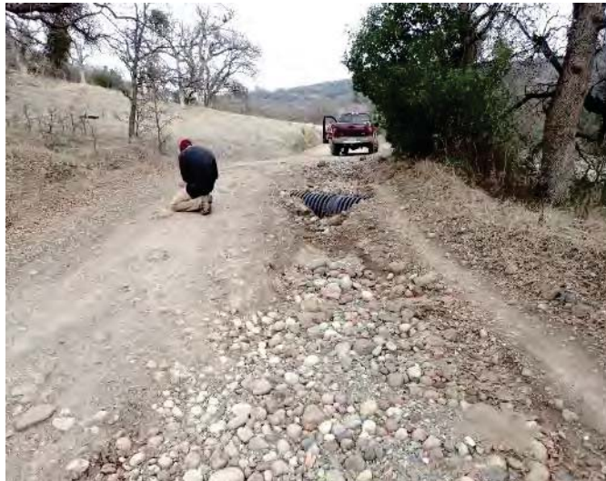
Figure 2. At feature #27 the stream crossing culvert is exposed by erosion cause by an active road surface gully.
