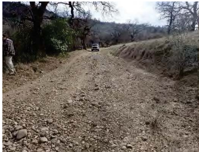
Figure 8. On Upper Park Road a berm has formed after years of grading and road surface erosion. The berm captures and concentrates road runoff, preventing it from being dispersed onto the hillside, and accelerates road surface and ditch erosion rates.
