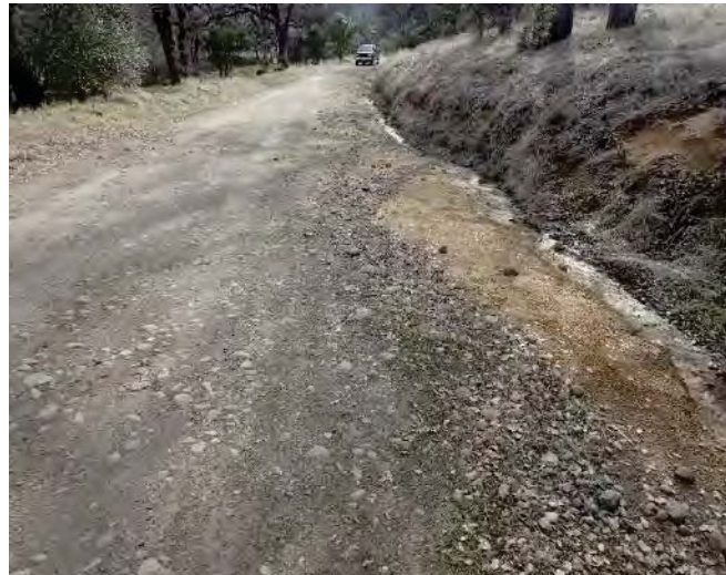
Figure 6. Road surfaces, berms and ditches capture and transport hillslope runoff and direct rainfall during storms. Road surface and ditch runoff often flow down the road grade and directly into stream crossing culvert inlets.
