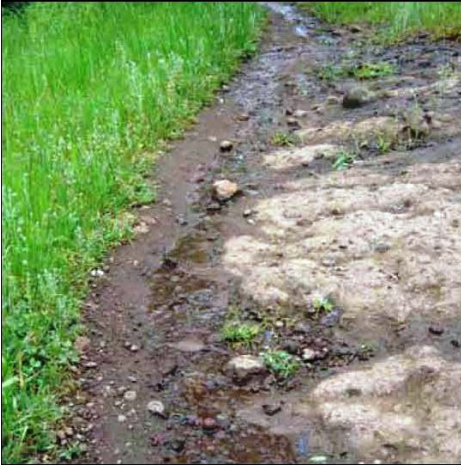
Photo 1 - Drainage running down trail causes users to venture uphill of the trail, creating soil erosion and trail widening. Installation of drainage controls are needed.
