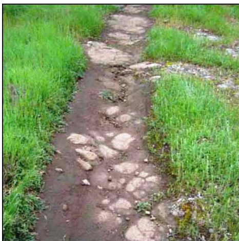
Photo 11 - Trail is functioning as a drainage conveyance, eroding soil to expose rock.
