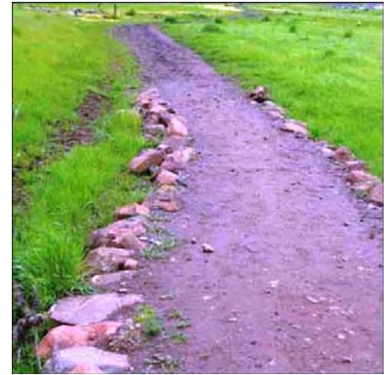
Volunteer and City constructed trail edge border near Horseshoe Lake is successfully controlling path width.
