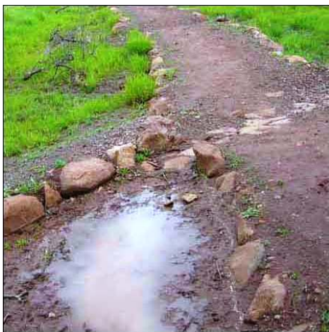
Photo 17 - Improperly installed dip is creating a low point for drainage problems.
