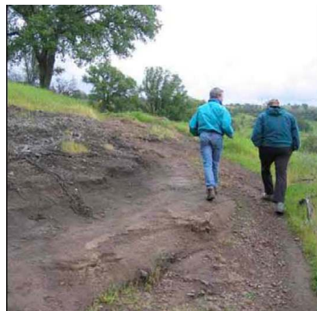
Photo 15 - Even use of erosion matting has been unsuccessful in maintaining soil on this trail. Reconstruction and low barriers may help contain soils and users here.
