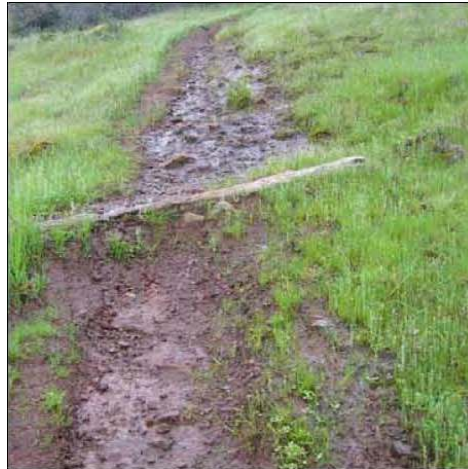
Photo 20 - Improperly installed log water bar on a mountain bike unofficial trail.
