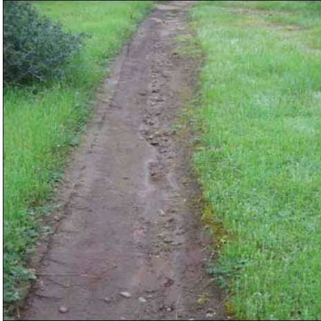
Photo 2 - No drainage conveyances are installed and water is running directly down the trail alignment.
