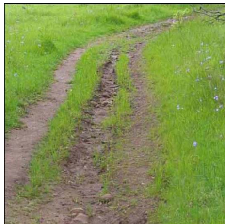
Photo 12 - Original trail in center has become rutted, causing users to create other paths which are easier to navigate and usable when water runs in the center path.
