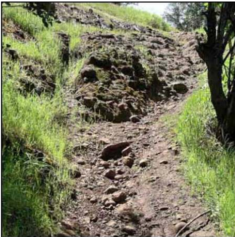
Photo 22 - Steep, eroded trail on the south rim. Steps should be installed or the trail should be re-routed.
