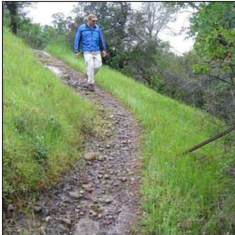
Photo 5 - No drainage conveyances are installed and water is running directly down the trail alignment. Rock is beginning to become exposed.
