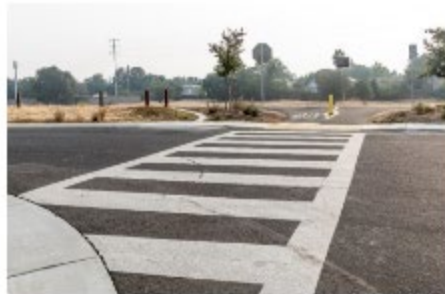
High Visibility Markings
