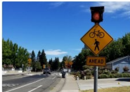
Signs and/or pavement markings that give motorists advanced warning of a crosswalk ahead
