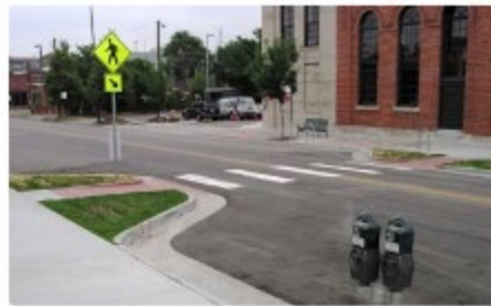
Curb Extensions (also known as bulb-outs) that shorten the crossing distance for pedestrians and improve visibility and encourage drivers to slow down due to the visual and physical narrowing of
