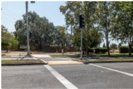
Pedestrian refuges (protected spaces in the center of the road on wide streets with long crossings)
